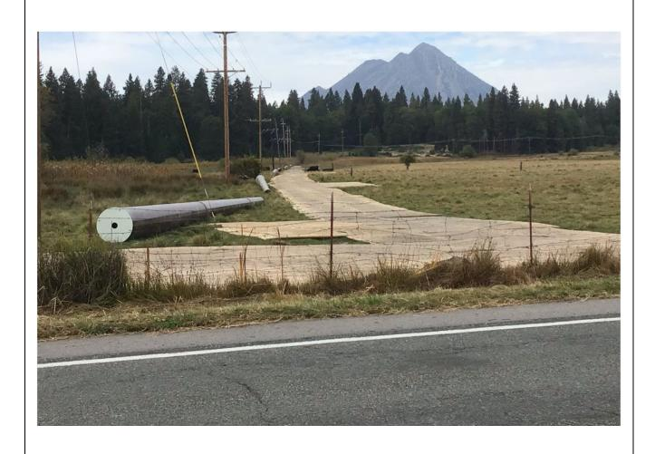
**Photo 2:** Poles were observed staged along the ROW north of Hatchery Road. Timber mats were installed in accordance with APM-BIO-5.
